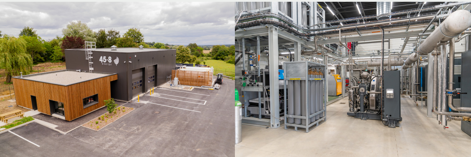
View of the helium pilot production unit located in the French Nièvre department
